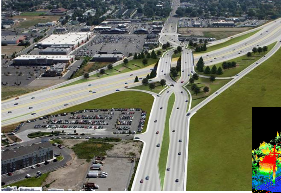
Left: Diverging Diamond Interchange on I-15 at Pioneer Crossing in American Fork, UT
