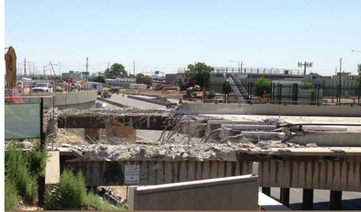
The old Pecos bridge during demolition. (Photo courtesy of Wilson & Co.)
